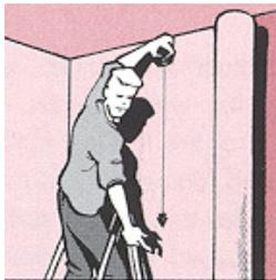
The **plumb line** will show whether the Jacquard pattern is straight. Use the plumb line again after each recessed or protruding corner.
