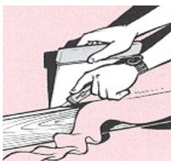
Using a spatula, press the textile to the wall and trim at the floor. Using a **sharp blade**, cut away all surpluses of fabric along the edge at the spatula. **Renew the blades regularly !**
