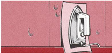
Small air bubbles can occur on a poorly prepared surface. Smooth these out using an iron **set to cotton**. Place a **clean sheet** between the iron and the wall coverings. If the wall covering does not stick, there is not enough adhesive.
