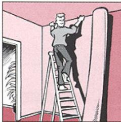
Leave the adhesive for a few minutes if the surface is non-absorbent. This increases adhesion and prevents the adhesive from seeping through the product. Press the wall coverings onto the adhesive in an upper corner. Roll out approx. 3ft (1m) and position the roll at an angle to the wall.
